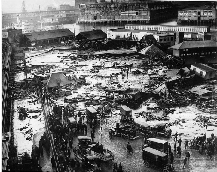
Figure 1. Aftermath of molasses tank failure
