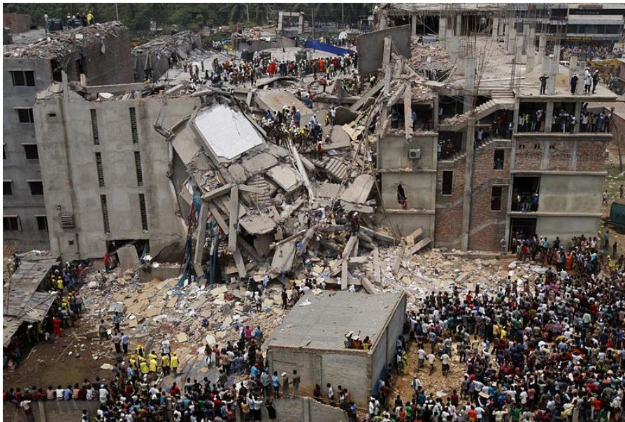
Figure 2. Aerial view of collapse.
